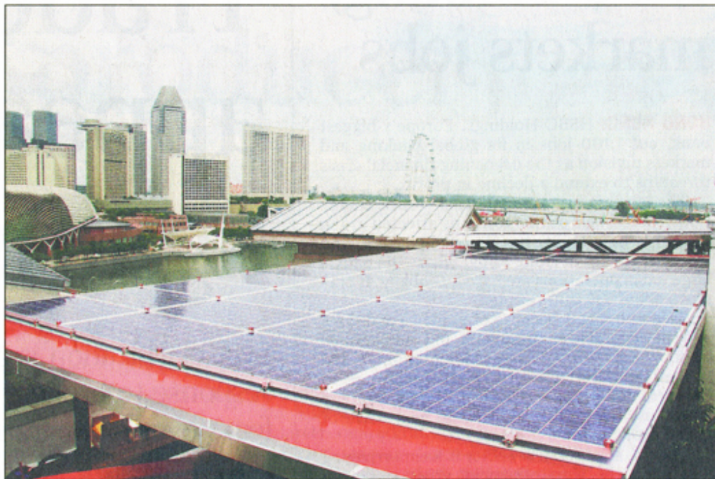
Singapore FreePort has installed a solar canopy on top of its skylounge hospitality suite at the Fullerton Hotel to offset carbon emissions this weekend. PHOTO: SINGAPORE FREEPORT
